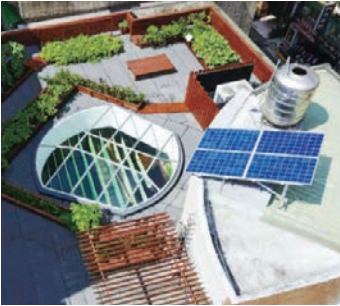
"Ecological hydroponic green rooftop from solar power generation and rainwater harvesting systems"
